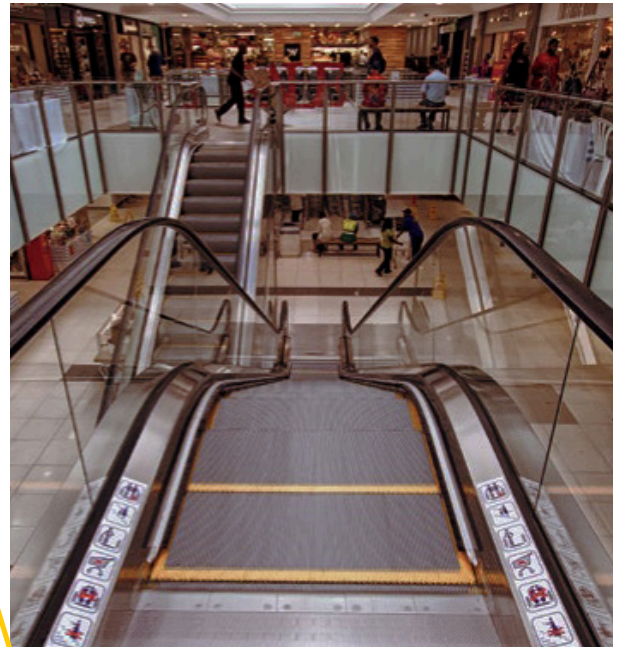
I'LANGA MALL • Client: Resilient Property Income Fund Description: 2 Escalators, 4 Goods Lifts and 1 Observation Lift
