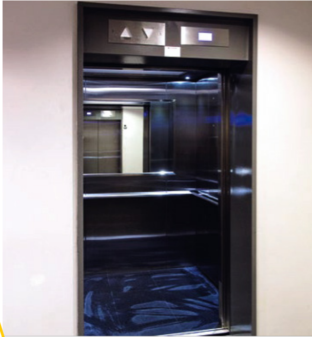
DID Hospital Upgrades • Client: Department of Infrastructure and Development Description: Replacement of 22 Elevators in 5 different hospitals
