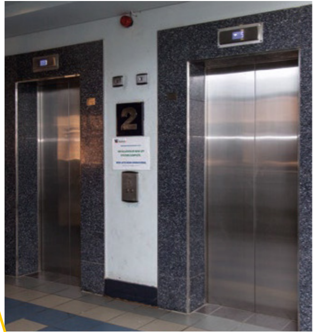
Kempton Park Civic Centre • Client: Ekurhuleni Metropolitan Municipality Description: Replacement and Upgrade of 9 Elevators
